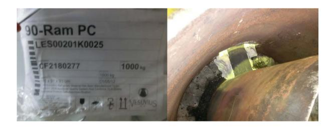
Carbon lining paste us used to finish up the bottom lining. The lining should be compact just as the firs layer of bottom lining. Use a rod, or a hammer, or your feet to compress the lining material. Make sure that the bottom is slightly tilted towards the tap hole, and that the bottom
