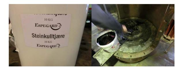
The bottom lining\electrode is made of carbon cold lining
