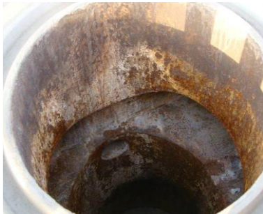
Inner cavity erosion of RAM BOP
