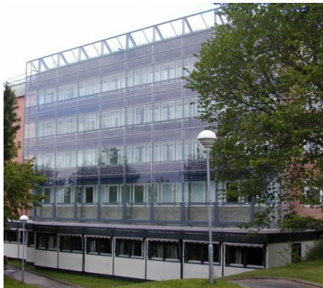
Figure 6. PV integrated in facade at Norwegian university of science and technology (NTNU)
