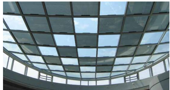
Figure 25 Semi-transparent PV integrated on roof_ elementary school in Munich- Trudering (Germany)
