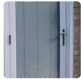
Figure 10. Venetian blind between glazing
