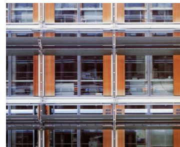
Figure 17. External shading system (SOKA-Bau – Wiesbaden)
