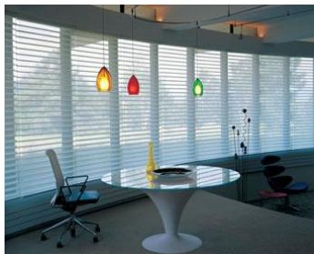
Figure 8. Internal shading- venetian blinds
