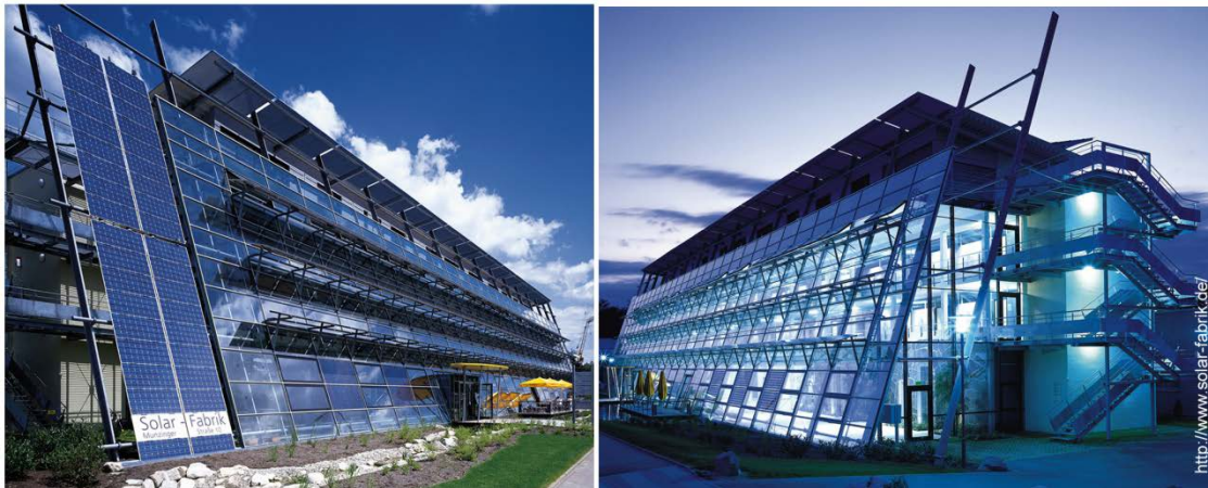
FIG 4.13: Inclined PV integrated façade of Solar-Fabrik building, Freiburg, Germany
