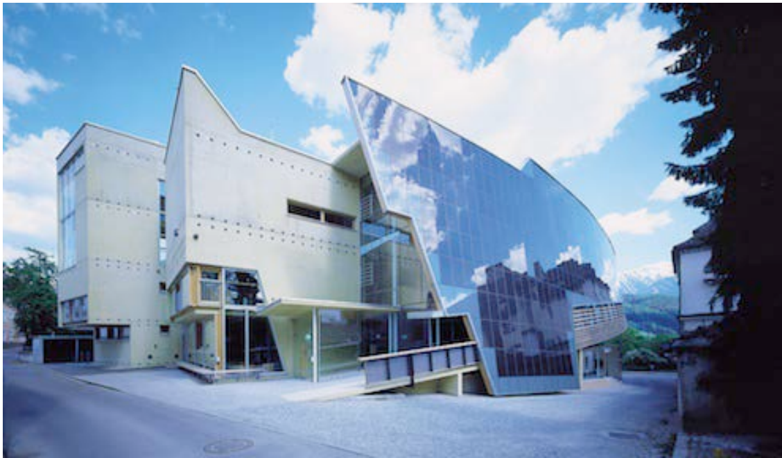
FIG 4.12: Inclined PV integrated glazed façade of Vocational College in Tirol, Austria
