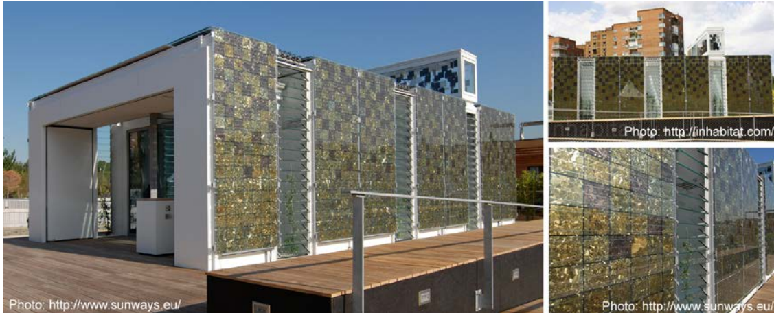
FIG 8.4: Multi-crystalline PV system with bronze and gold coloured silicon solar cells used in the "home+" building project submitted by Stuttgart University of Applied Sciences,
