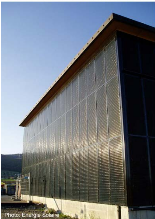
FIG 9.6: Façade integration of unglazed flat plate collectors as multifunctional cladding element, (CeRN), Switzerland.
