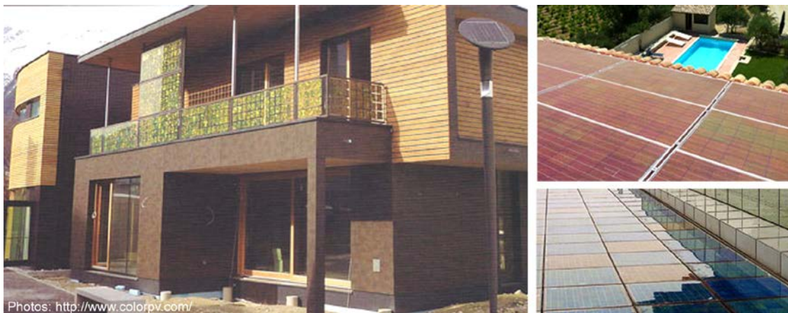
FIG 8.3: (Left): PV modules based on Metallic Gold cells are integrated in the balcony, rails and facade, Tirol, Austria
