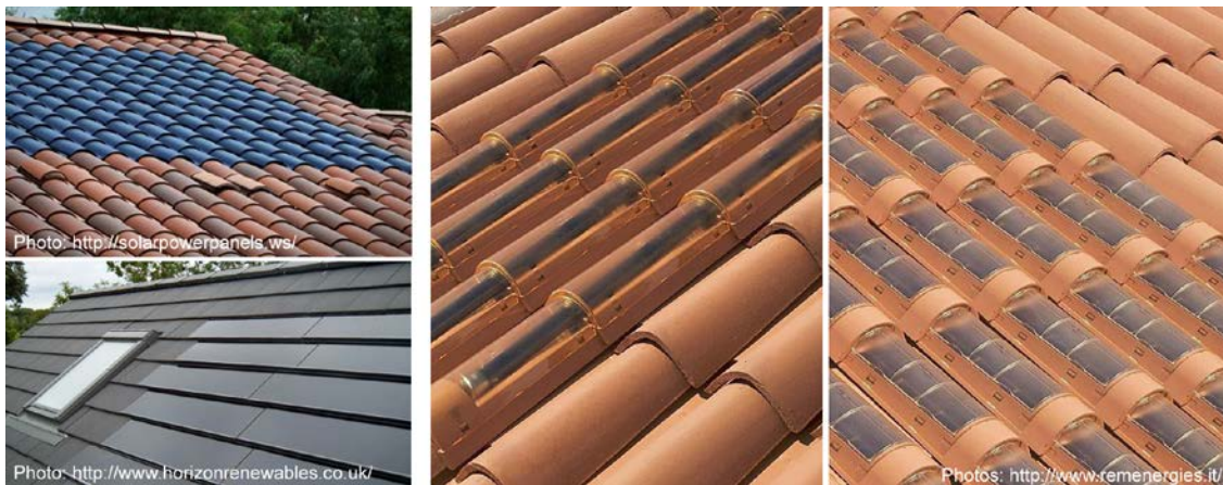
FIG 8.1: (top-left): PV tiles on the roof, (bottom-left): PV on the roof Delamont Country Park Ireland building, (center & right): Techtile Therma STC systems on the roof
