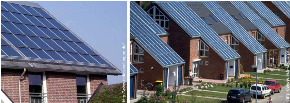
FIG 5.3: Integrated STC systems in Hamburg Bramfeld multi-family house, Germany
