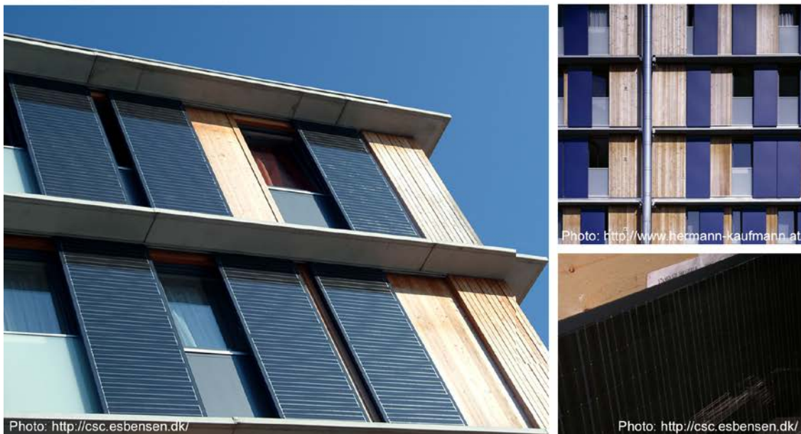
FIG 9.3: Integration of thin-film PV on the sliding sunshading, Dwelling houses Spinnereistraße, Austria,
