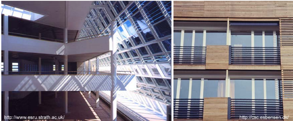
FIG 6.1: (Left) Integration of PV as shading and daylight control; (Right) Evacuated Tube collector used as balcony railing
