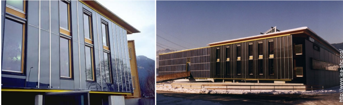
FIG 5.4: Integrated STC systems on the façade of office building of AKS DOMA Solartedhnik
