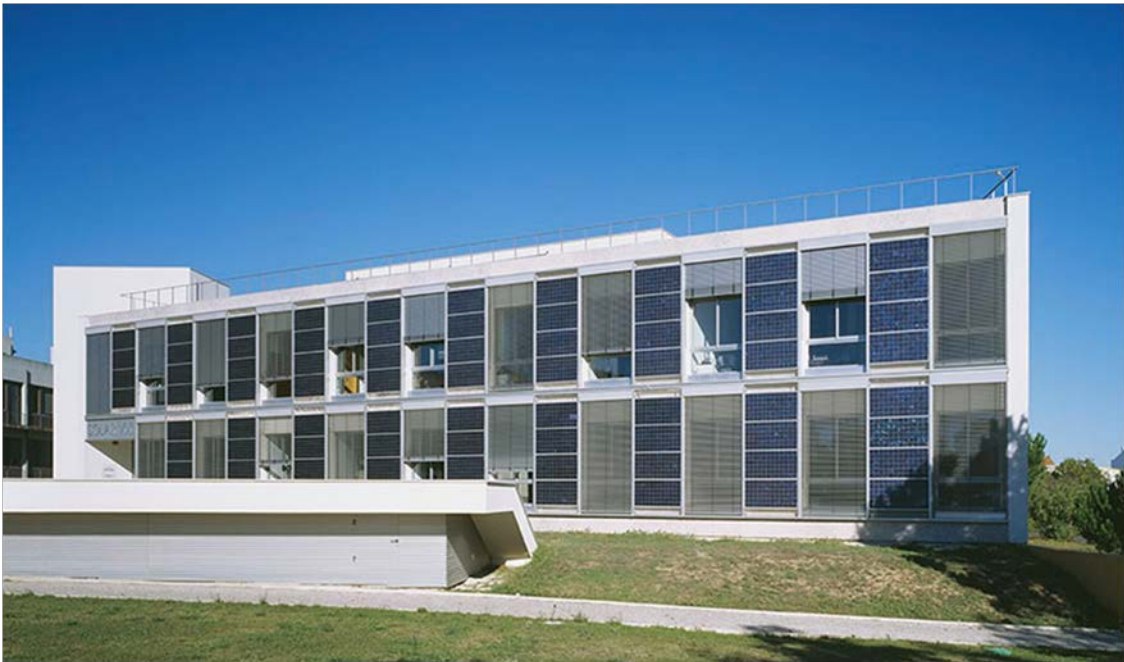
FIG 4.9: PV integrated into the opaque parts of the façade of Solar XXI building, Portugal
