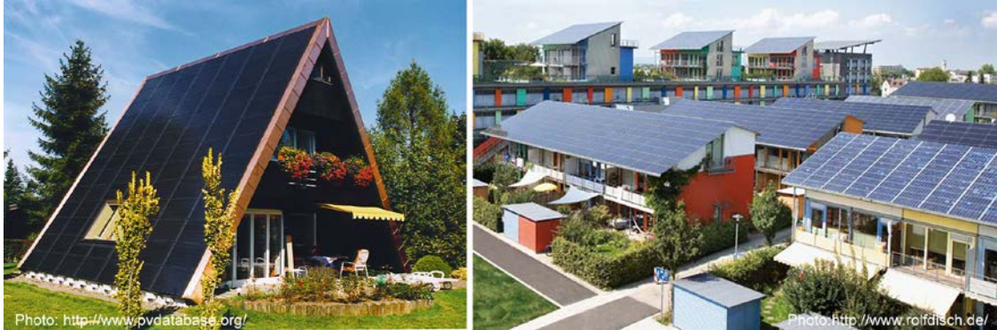
FIG 4.4: (Left) Integrated PV on the pitched roof of vacation house Bartholomä-Park in Germany (Right) Integrated PV roofs in Schlierberg Solar Settlement in Freiburg Credit: http://www.pvdatabase.org/ , http://www.rolfdisch.de/
