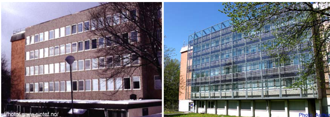
FIG 3.2: (Left) Office building at NTNU before PV integration, (Right) Same building after PV integration on the glass façade
