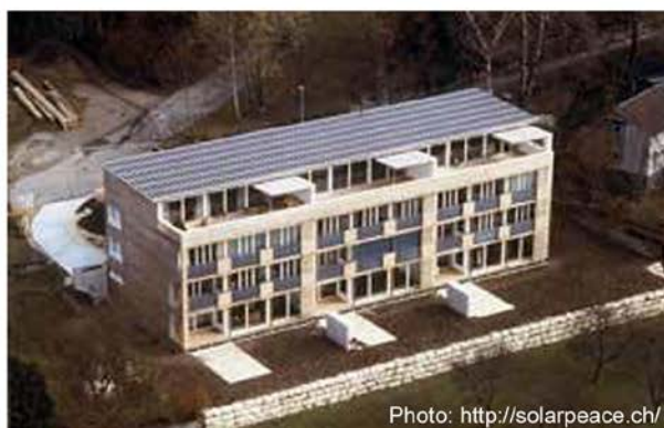
FIG 9.5: Integration of evacuated collectors as balcony railings, Sunny Woods, Switzerland
