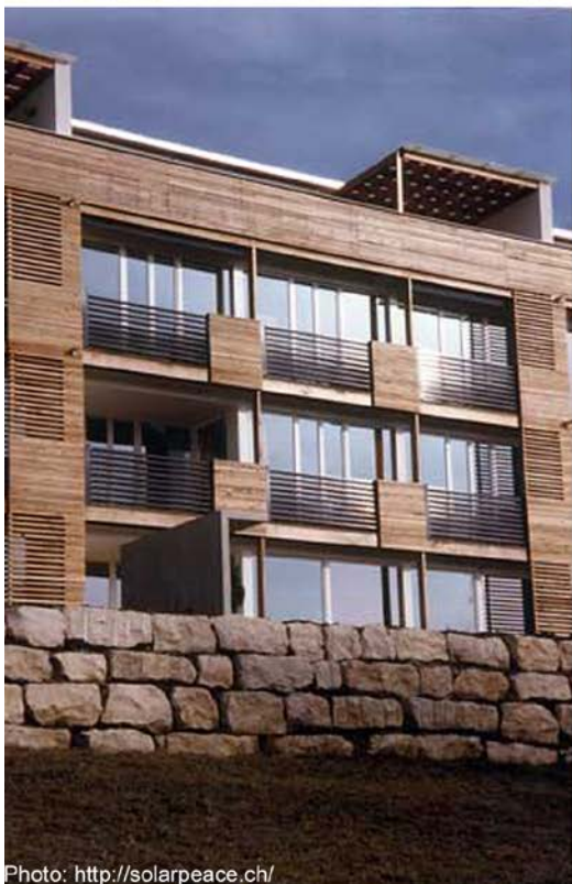
FIG 9.5: Integration of evacuated collectors as balcony railings, Sunny Woods, Switzerland
