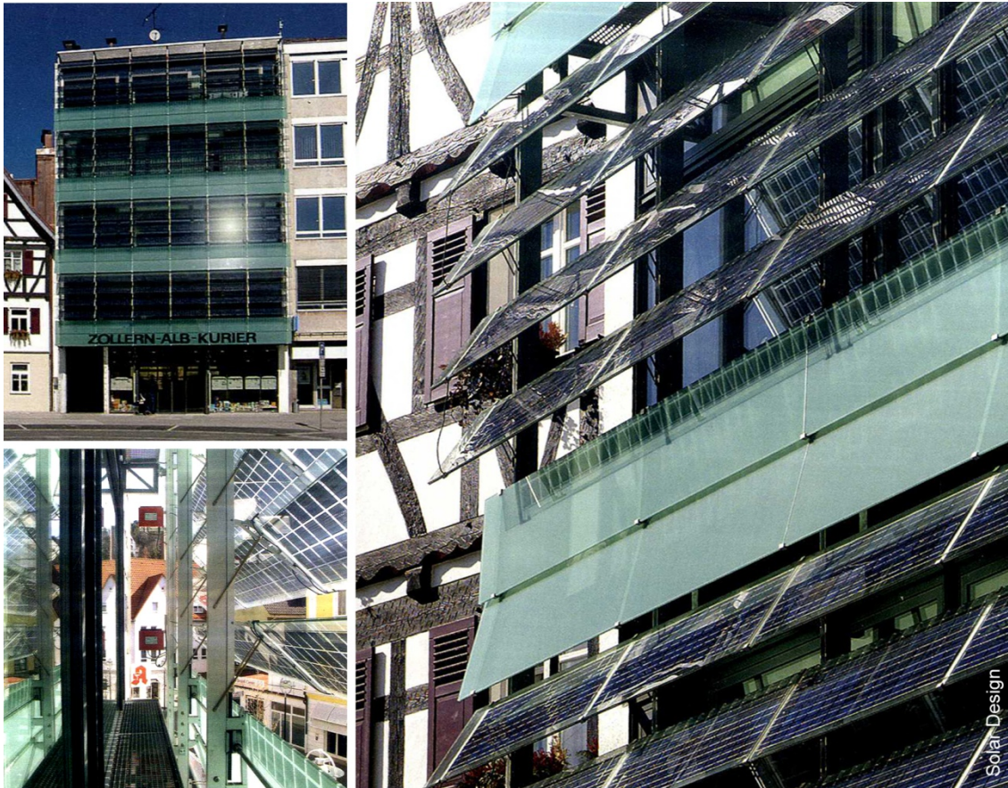
FIG 4.16: PV integrated into the glass louvered sun-shades in the Editing office, Albstadt-Ebingen, Germany Credit: Solar Design
