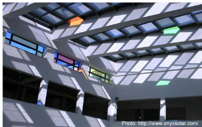
FIG 4.8: (Left) Atrium with PV modules, Ludesch/Vlbg., Austria; (Right) PV on coloured skylights at Bejar Market, Salamnca, Spain
