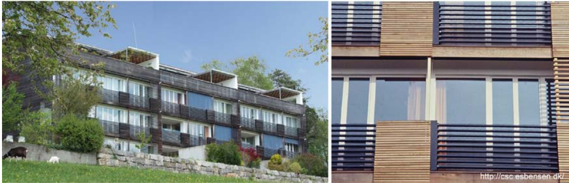
FIG 5.6: Use of evacuated tube collectors as balcony railings, Sunny Woods multi-family housing in Zurich, Switzerland
