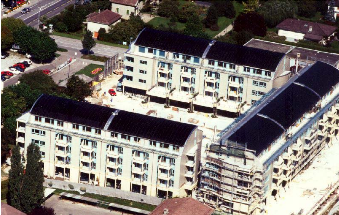
FIG 3.1: Elegant use of solar thermal collectors on the curved roof of 'Solar City', housing development in the suburb Plan-les-Quates, Switzerland
