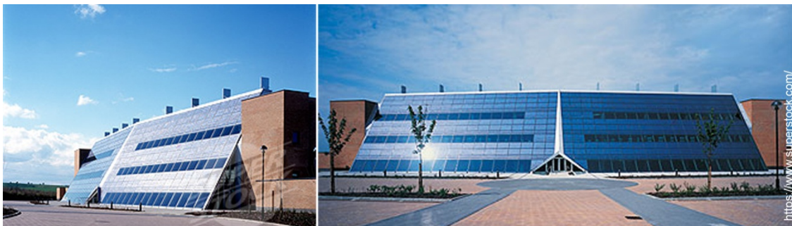
FIG 4.14: PV integrated inclined wall of Daxford Solar Office
