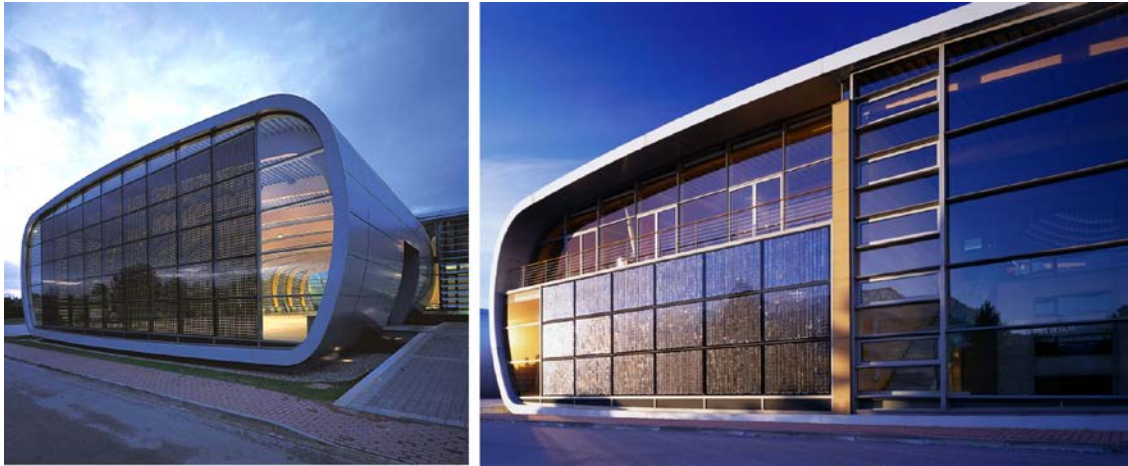
FIG 4.10: Tobias Grau Production Building in Germany has PV integrated into its south glazed facade
