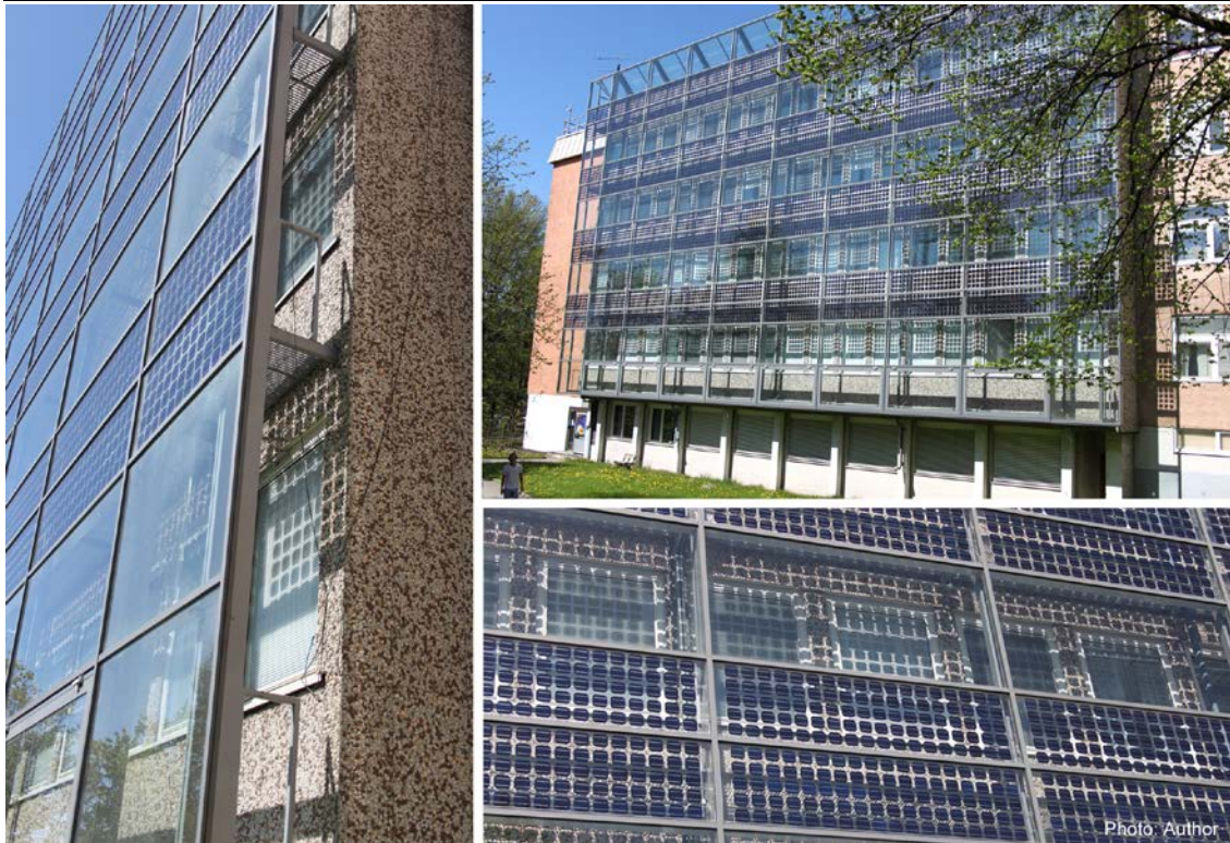
FIG 9.1: Mono-crystalline PV cladding on the glass façade, BP Solar building, NTNU, Trondheim,
