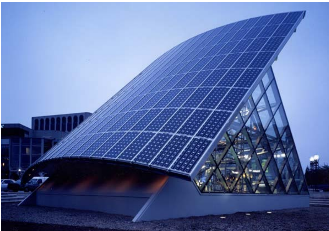
FIG 4.7: PV integration on the curved roof of BP solar Showcase in Birmingham Credit: http://www.solartechnologies.co.uk/
