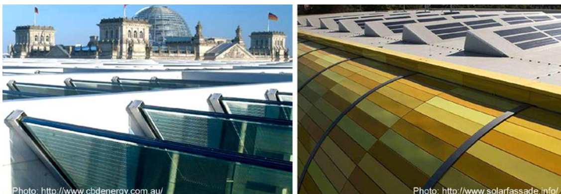
FIG 4.6 (Left) Integrated PV on the saw-toothed glass roof of Paul Lobe Haus, Berlin (Right) Sawtooth roof with PV integration, DIY store, Hamburg
