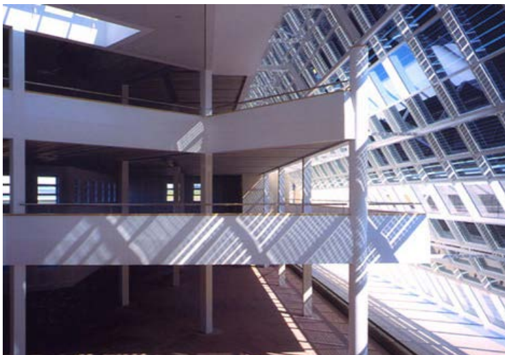
FIG 2.3: Doxford Solar Office Credit: http://www.studioe.co.uk/
