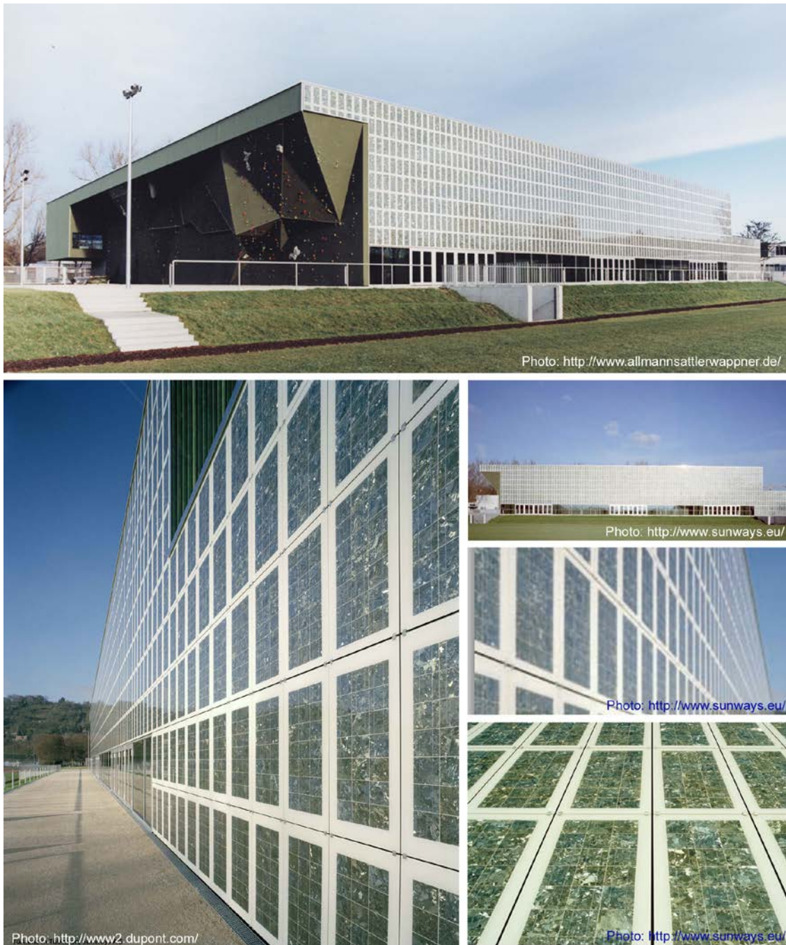
FIG 9.2: Integration of coloured poly-crystalline solar cells, Paul Horn Arena, Tübingen Germany
