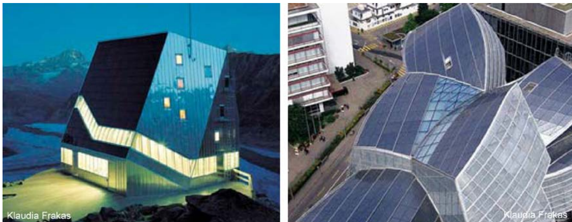
FIG 6.3: Integration of PV, considering the formal aspect. (Left) Monte Rosa Hut, (Right) Novartis Building, Switzerland
