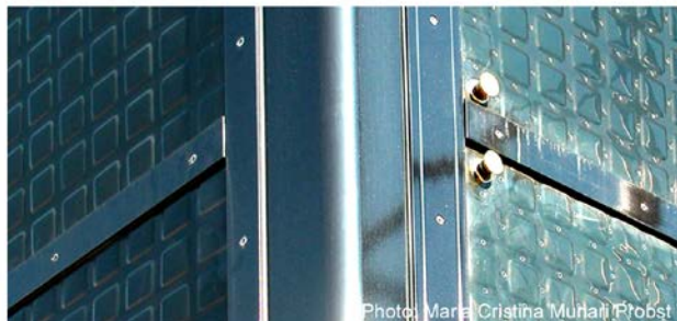
FIG 9.6: Façade integration of unglazed flat plate collectors as multifunctional cladding element, (CeRN), Switzerland.
