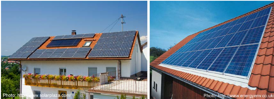
FIG 4.3: (Left) PV modules added on to the roof as pure technical element, (Right) Semi-integrated PV modules on the Roof
