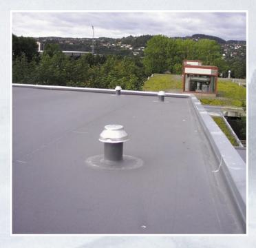
ently strong to transmit the wind suction forces from the roof. It is also possible for positive pressure to occur in individual buildings, which presses up against the roof from inside. The roof construction must be dimensioned to withstand these loadings, and this is an important condition for vacuum roofs.
