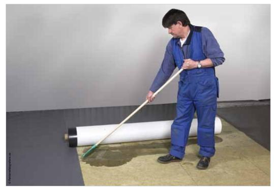
To secure the membranes against wind uplift, fully adhering is commonly used in countries where weather conditions favour installation.
