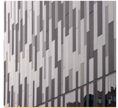
Fig.25 Photovoltaics in Combination with Stone and Glass (Lithodecor, Airtec system for ventilated curtain wall façades)
