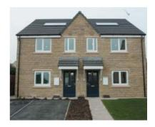
Some of the techniques that were used to make this sustainable homes include: solar panels, an air heat pump, water-saving measures such as controlled flow rate taps, improved U-values for the windows and external doors, and the use of Green Guide-rated materials.
