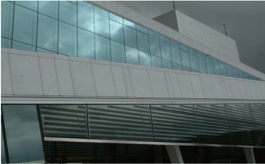
Opera House, Oslo, Norway
