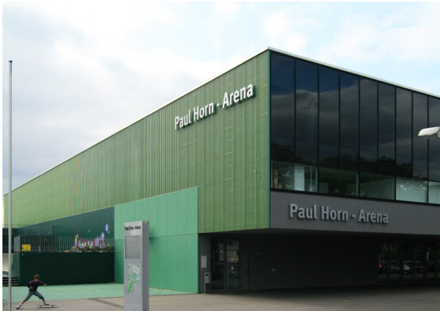
Paul-Horn Arena, Tübingen, Germany - Entrance
