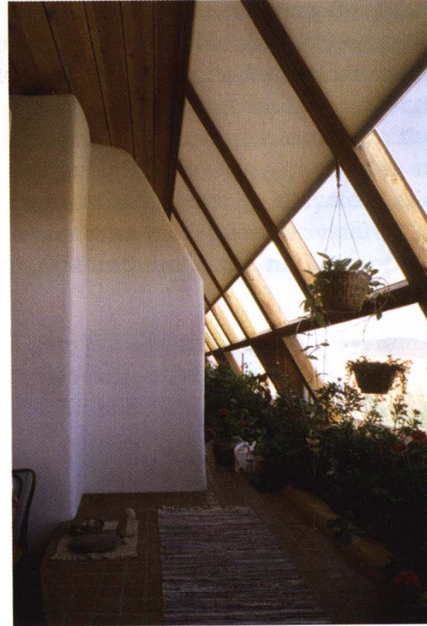
4.125 Classic example of solar apertures, solar control, and thermal mass in the Shaw residence in Taos, New Mexico.
