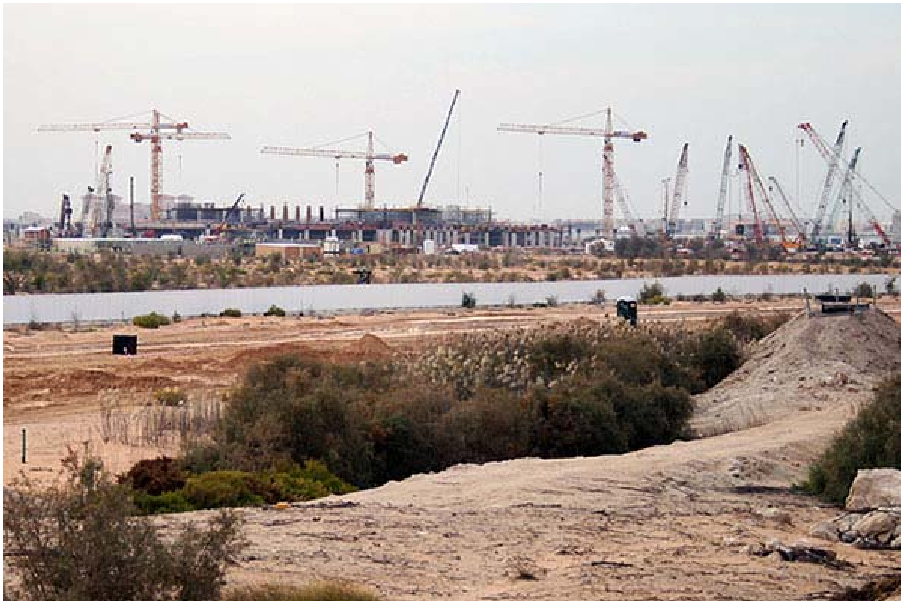
Masdar City is under construction – University scheduled to open in February 2010
