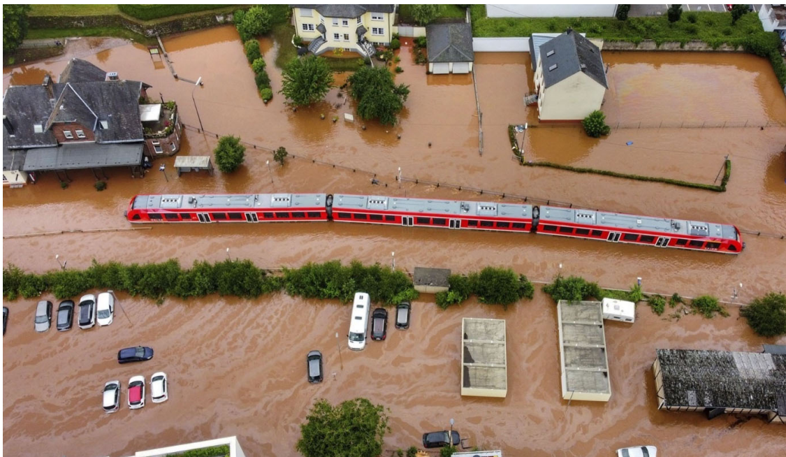
Fig.1. A regional train sits in the flood waters at the local station in Kordel, Germany, July 15, 2021.
