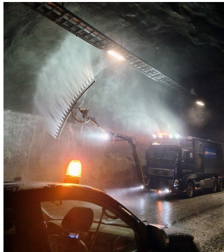
Washing of Grillstadtunellen (Trondheim), picture taken during sampling of wash water
