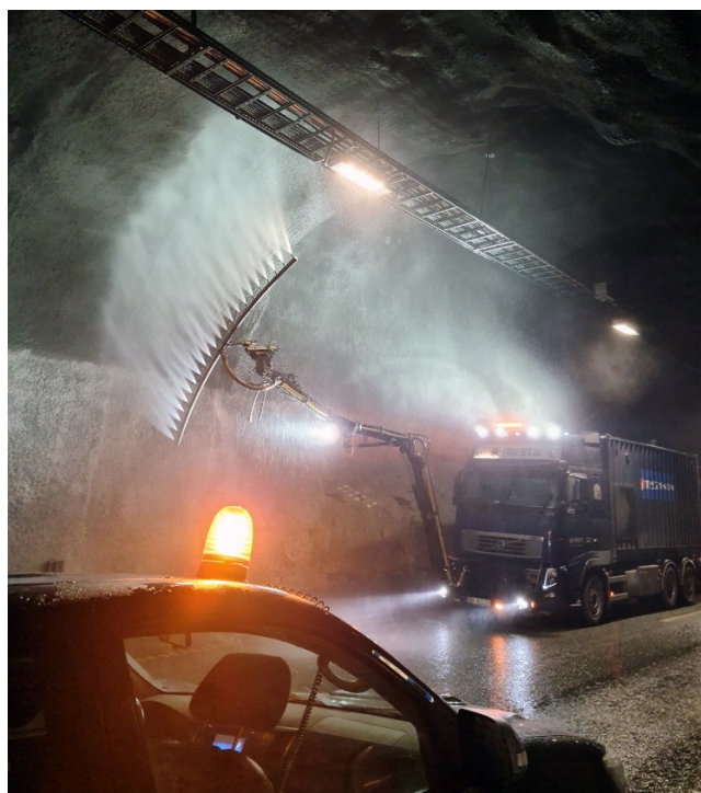
Washing of Grillstadunellen (Trondheim), picture taken during sampling of wash water
