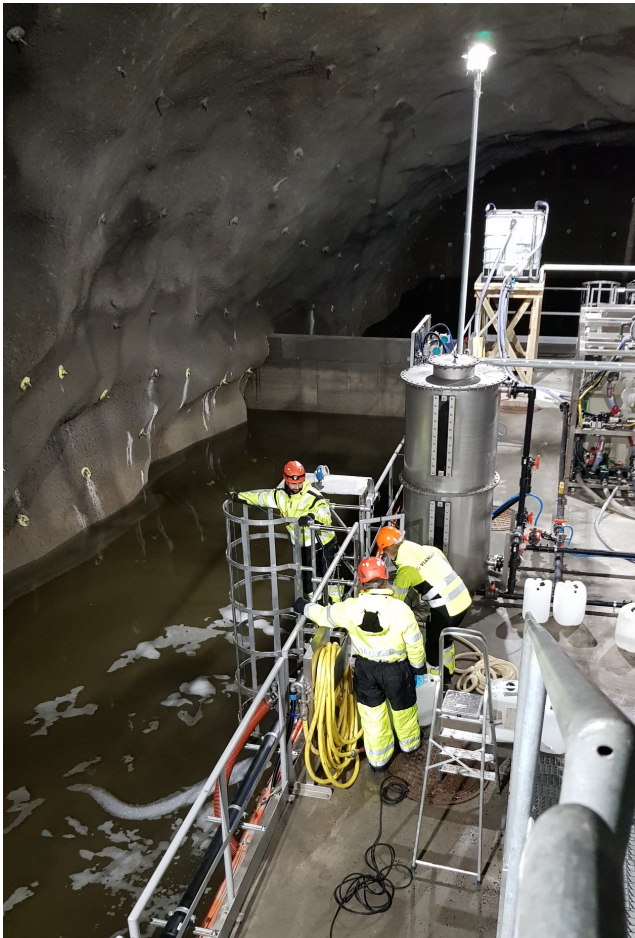
Sampling from a sedimentation basin at Bjørnegårdtunnelen (Sandvika)
