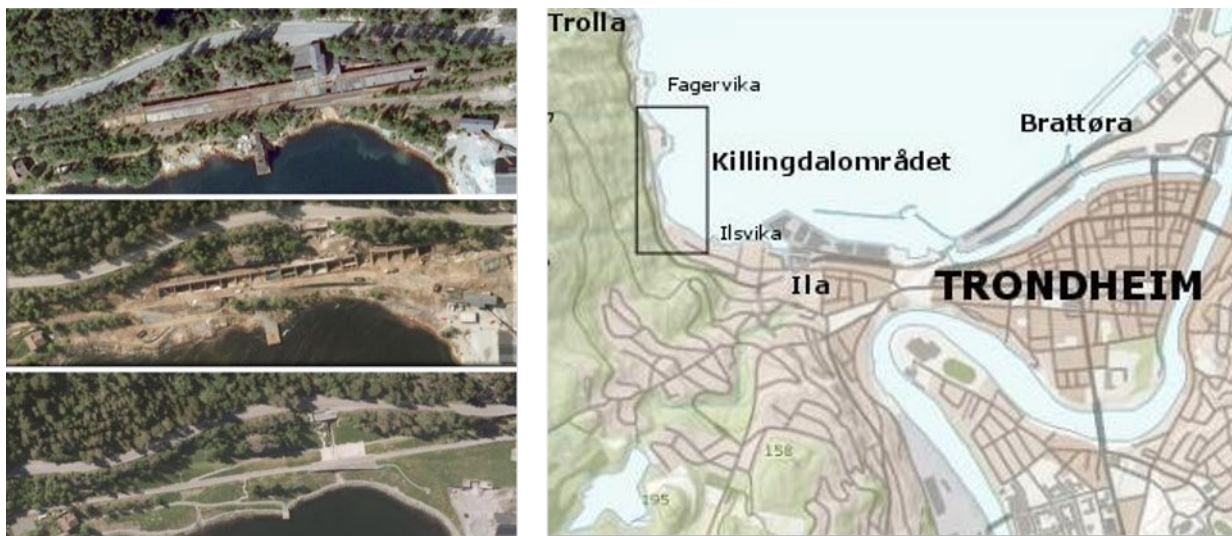
(Right) Aerial view of the Killingdal area: Before cleanup, during cleanup - the warehouse and unloading shafts are open and after finishing the project - new walkway and bike path follow the old railway tracks. (Left) Location of the Killingdal area in Trondheim.
