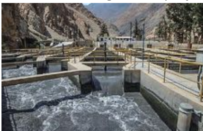
Desander facility at Cahua HPP, Peru www.hydropworld.com
