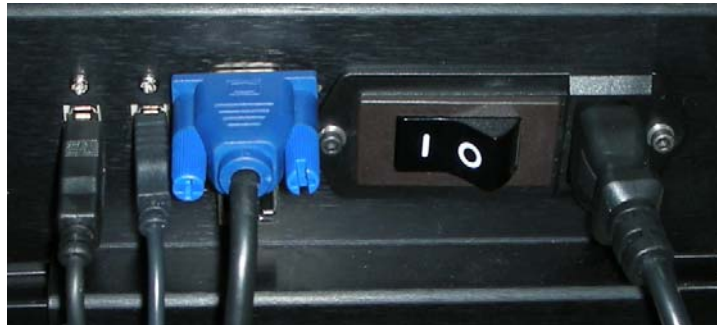
Figure 7-2: Main power cable and switch
