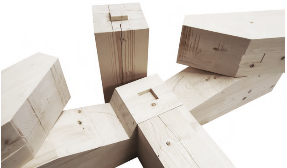
Detail 1 built in scale 1:1, pieces taken apart
