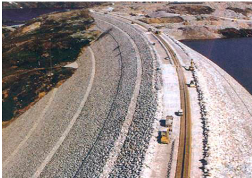
Example of a rockfill dam with riprap protection.
