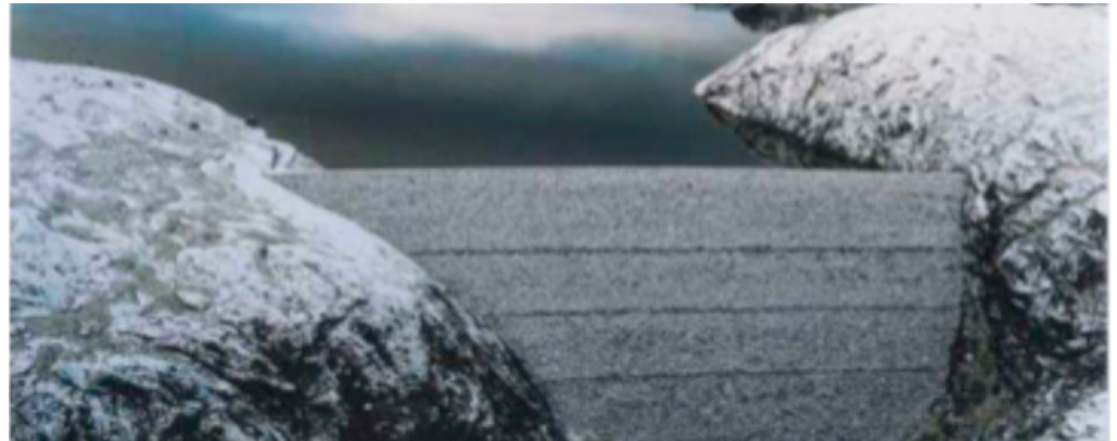
The rip rap at Dam Svartevatn
