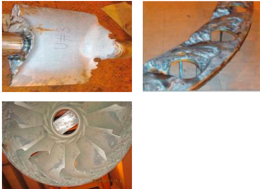
Sediment erosion in Francis turbine components
