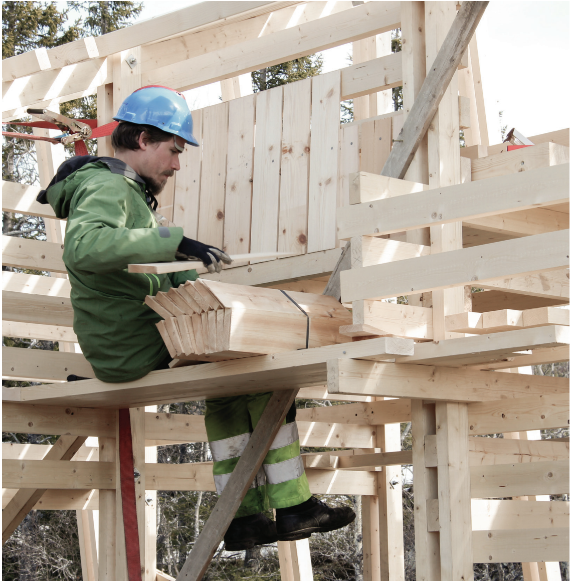
△ Wood shingles are used to cover parts of the western facade.
