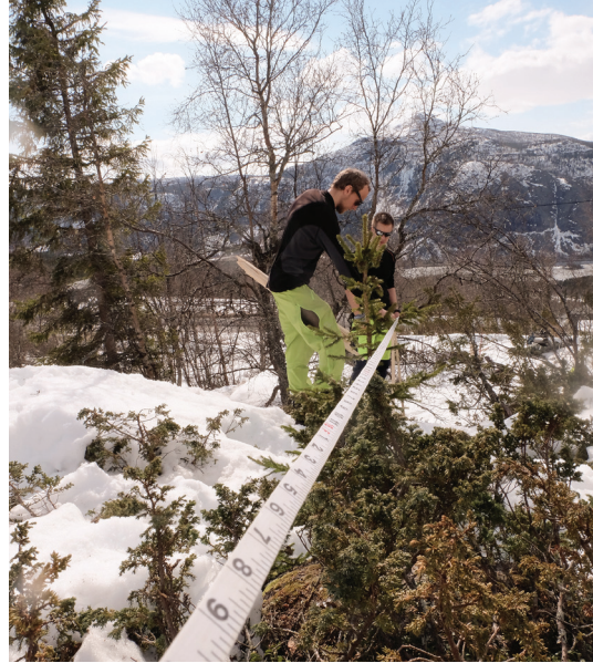
△ Measuring the site to find the foundation points.
