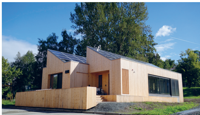
Figure 3. ZEB Living Laboratory. Main architect is Luca Finocchiaro, Faculty of Architecture and Fine Art, NTNU. Photo: Katrine Peck Sze Lim
