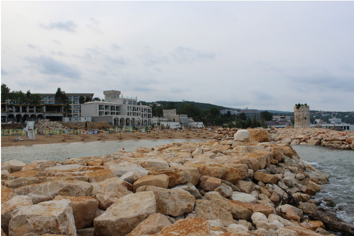
Figure 14. Varna coast, St. Konstantin and Helena Resort (Black Sea, eastern Bulgaria): modified marine habitats by recent constructions at the nearby seashores. Photo P. Michailova, 26.VI.2019.
