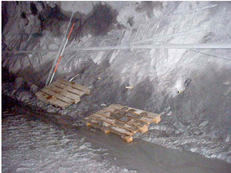
Figure 5: Position of three bore holes in the new tunnel.
