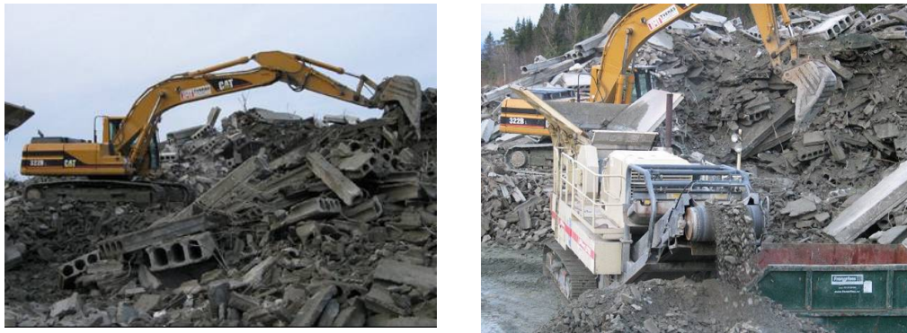
Figure 4: Material production; crushing and separation of reinforcement bars
