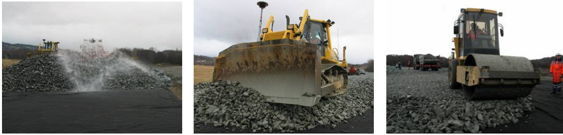
Figure 6: Sprinkling of crushed concrete materials is recommended before paving and compaction
