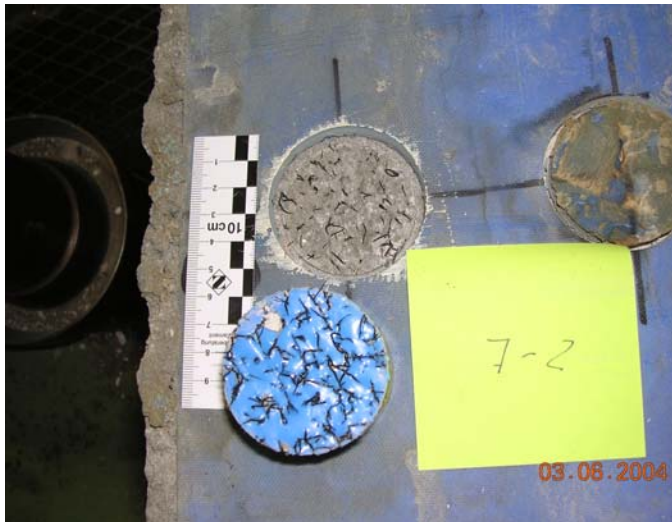
Figure 9: pull out test for the homologation of the fixation of the USP, according to the delivery conditions of DB AG
