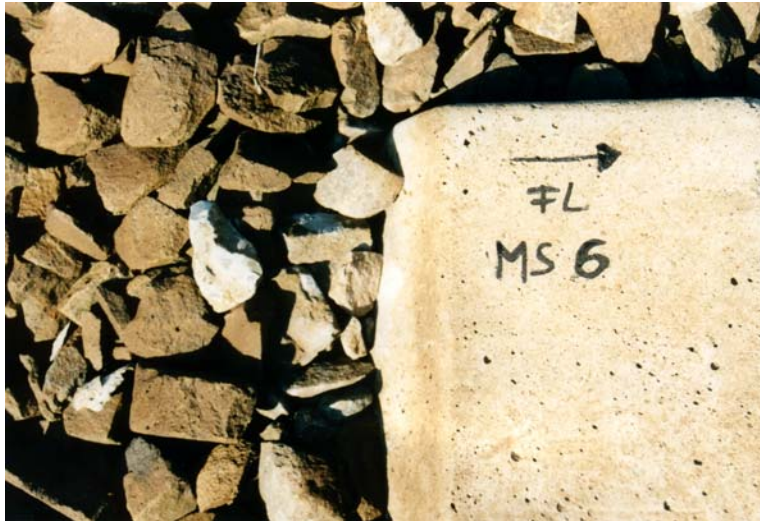
Figure 6: signs of abrasion of the sleeper flanks with USP
