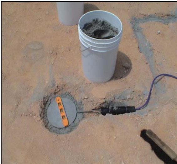
Figure 3b: Installation of earth pressure cell.
