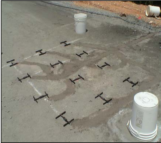
Figure 3a: Installation of asphalt strain gauge array.
