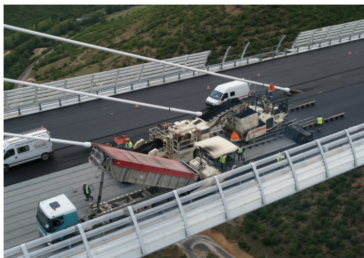
Figure 10: Laying Orthochape ® on the Millau Viaduct.
