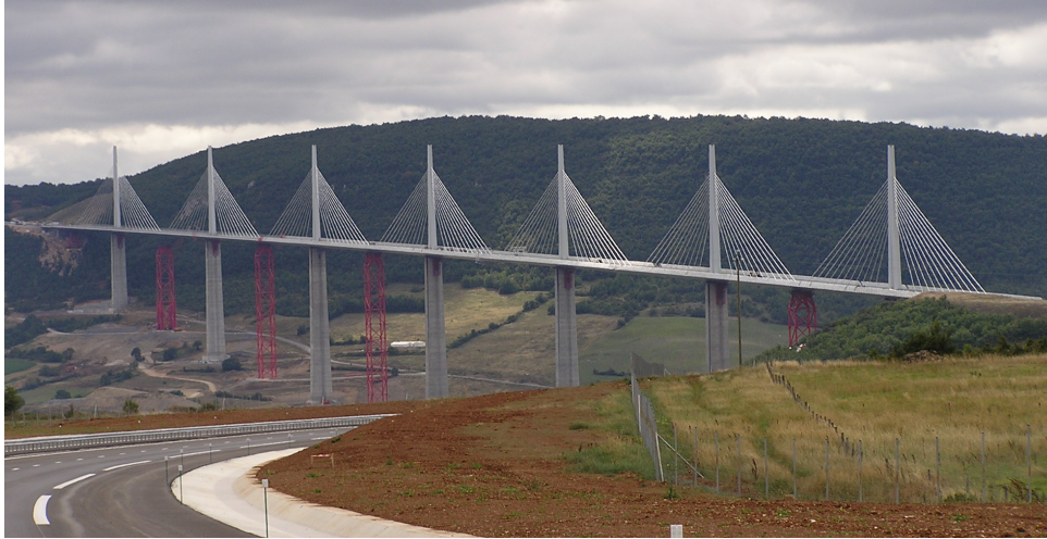
Figure1: Overall view of the Millau Viaduct.
