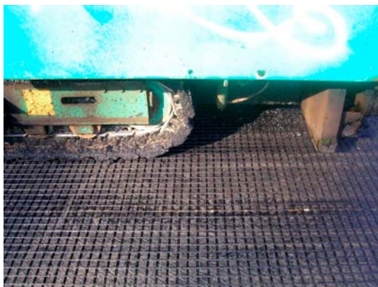
Fotograph 3: HaTelit ® C 40/17 trafficked by a tracked paver
