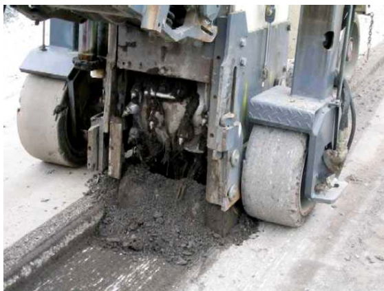
Fotograph 5: Milling of reinforced asphalt
