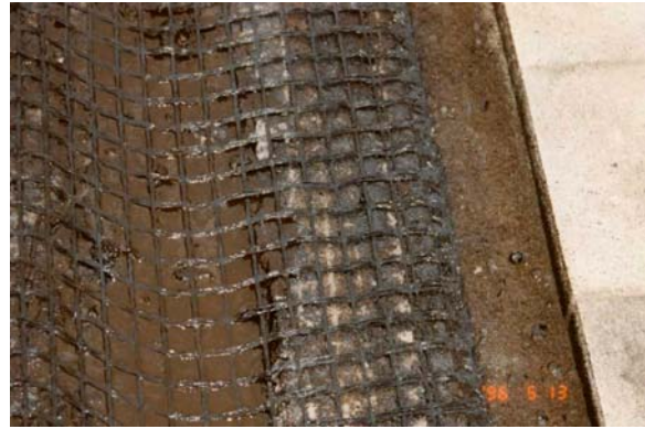
Fotograph 2: Difficult spots during installation
