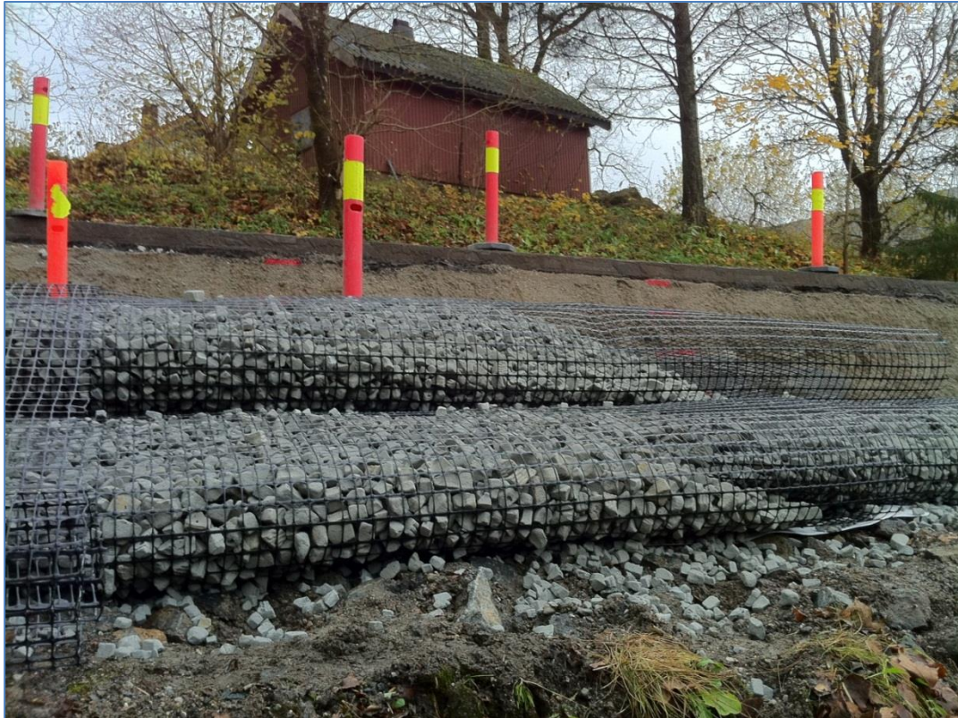
Figure 11: Mesh reinforcement around the foamglass [9] .
