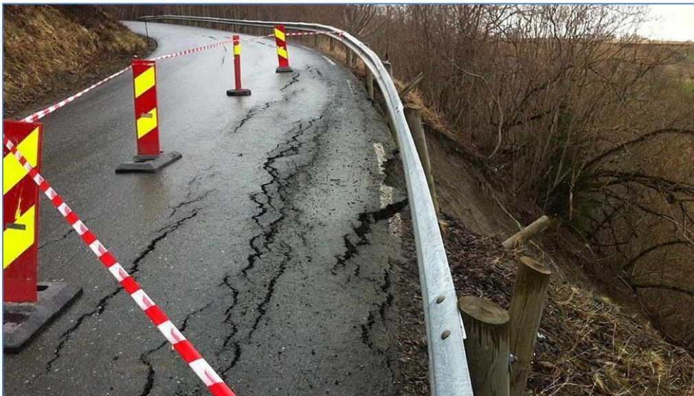
Figure 1: This picture is from Fv 734 (Varmbuvegen) in Melhus in Sør-Trøndelag [13] . It is a typical example of problems with instability in steep slopes and where it is large expectations regarding the method described in this paper. In Norway there is a large number of steep slopes with similar problems.
