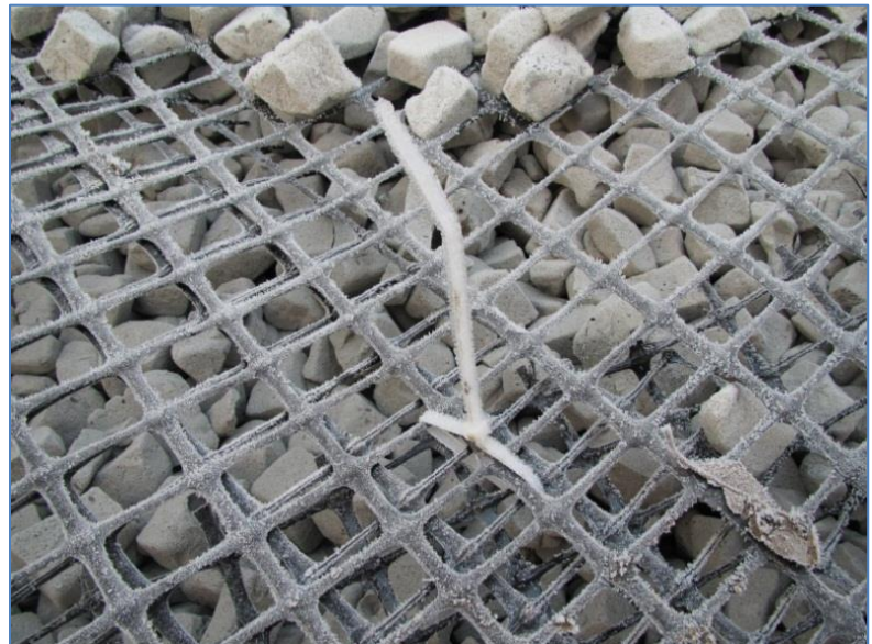
Figure 8: Geotextiles are joined with strips [14] .
