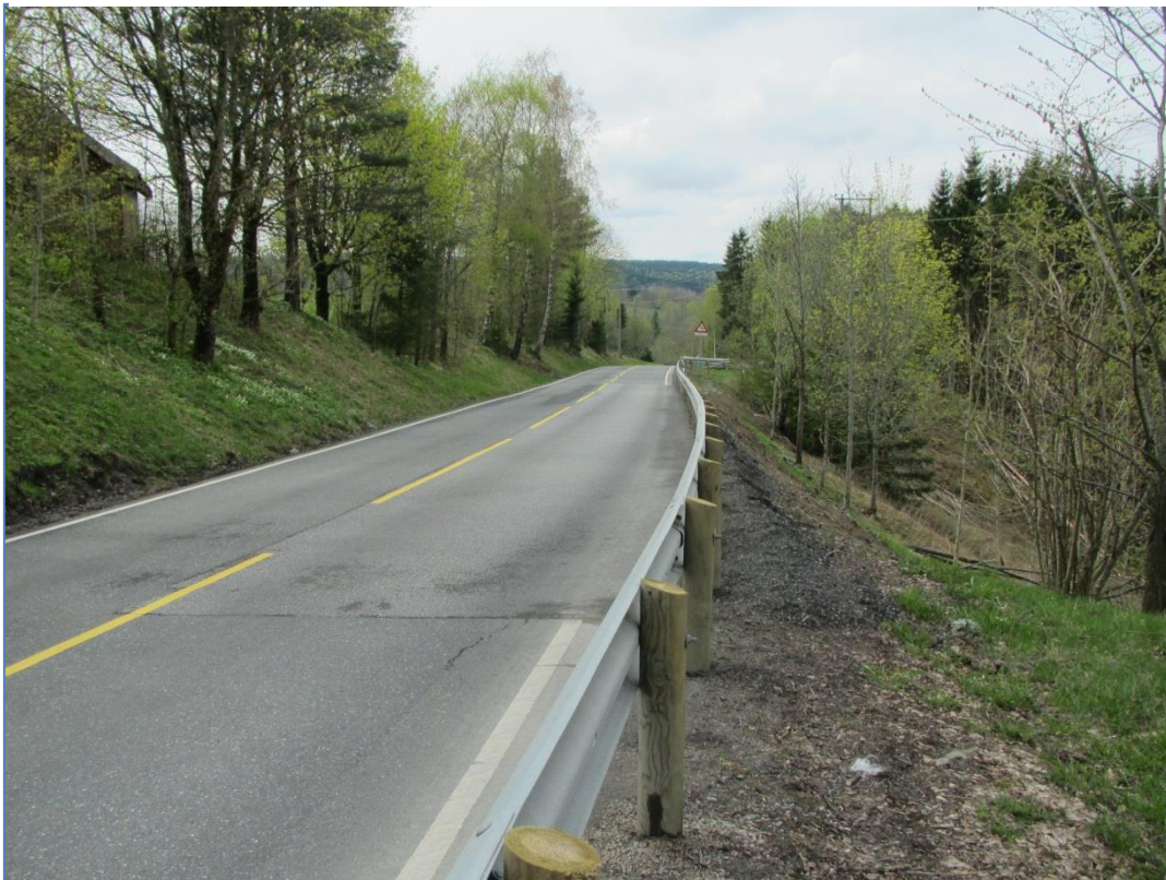
Figure 12: Same place as figure 2. Picture is taken 9 th may 2012 when the projectgroup was on inspection. 6 months after the first inspection there is no signs of deformation or settlements of the area that was repaired in fall 2011 [14] .
