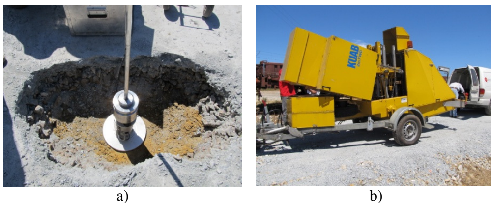
Figure 7: Load test equipment: a) LFD on the subgrade; b) FWD on the top of the reinforcement layer.
