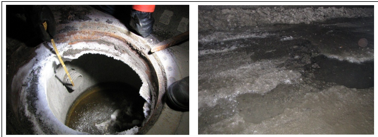
Figure 2: Shallow and frozen drainage well (left) and ice lump formation (right)
