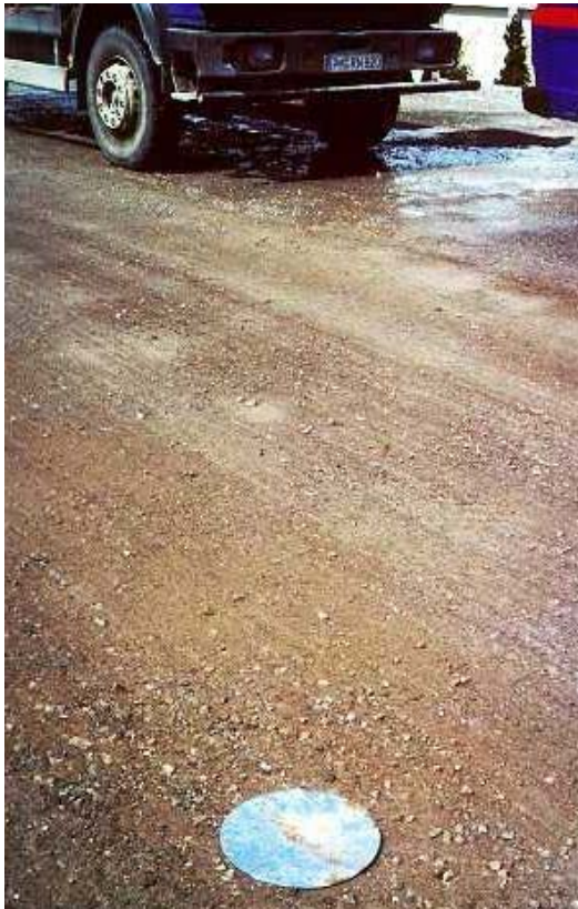
Figure 3: Unbound base layer with high bearing capacity but low permeability.
