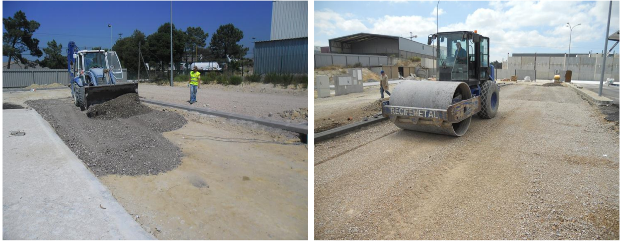
Figure 3: Construction of the experimental sections.
