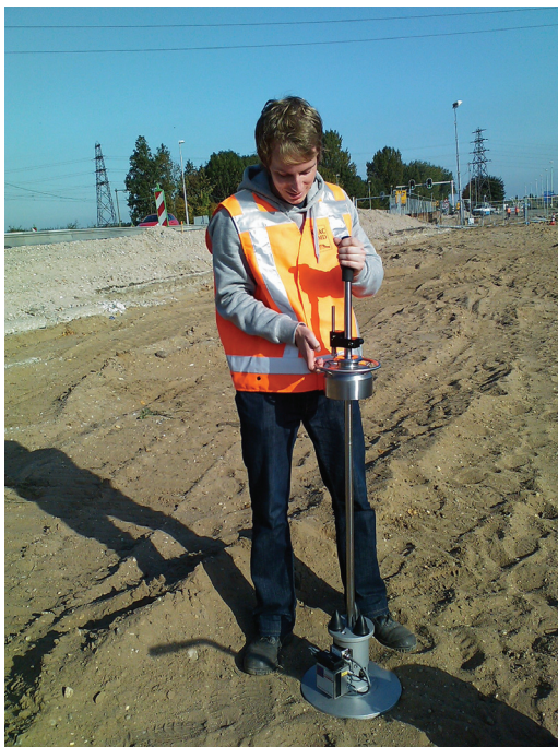
Figure 4: Light Weight Deflectometer test
