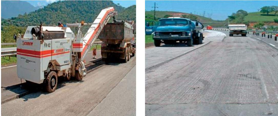
Figure 2: Miller and milling service on a road (Bernucci et al. , 2006).
