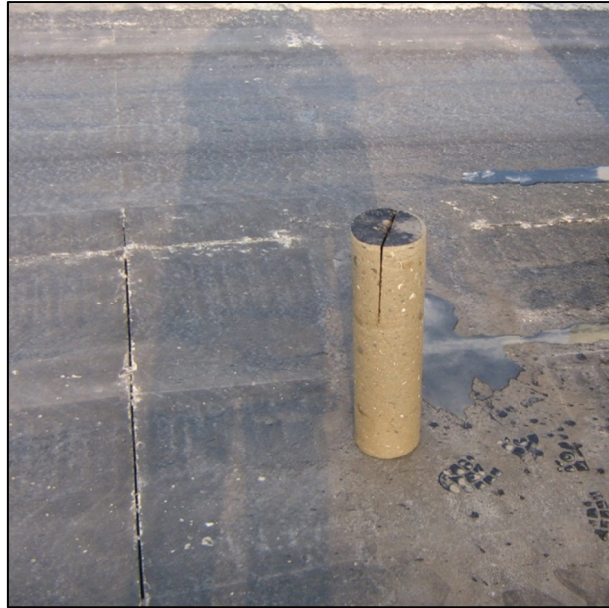
Figure 20: Core drilled at a notch in the CTB
