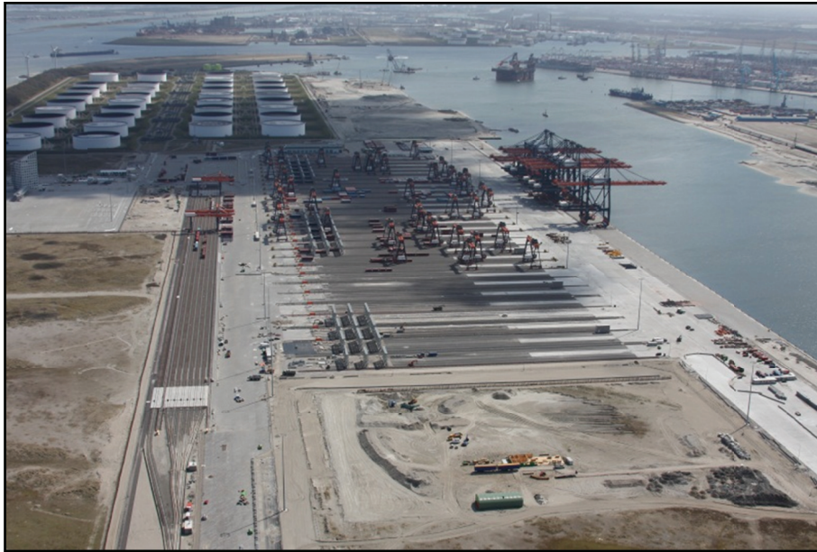
Figure 1: Overview of a part of the Euromax Container Terminal Rotterdam
