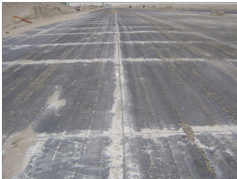
Figure 19: Notch pattern at the surface of the CTB
