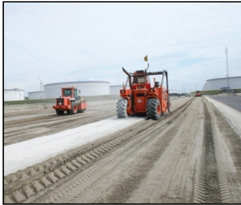
Figure 4: In-situ construction of Cement Treated Base
