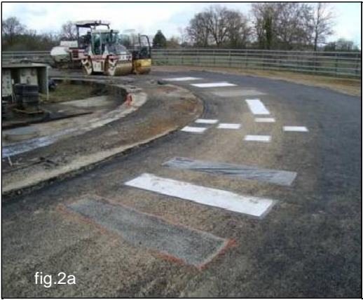
Figure 2. 2a: Interface defects before wearing course construction 2b: Map of the different debonded areas
