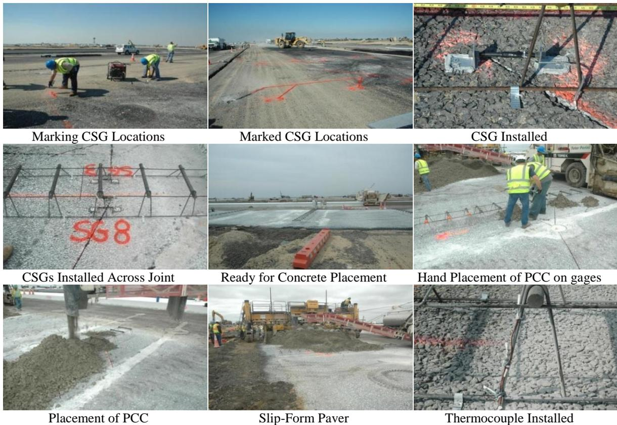
Figure 5: Installation of CSG and Thermocouple in Taxiway-Z pavement instrumentation project.
