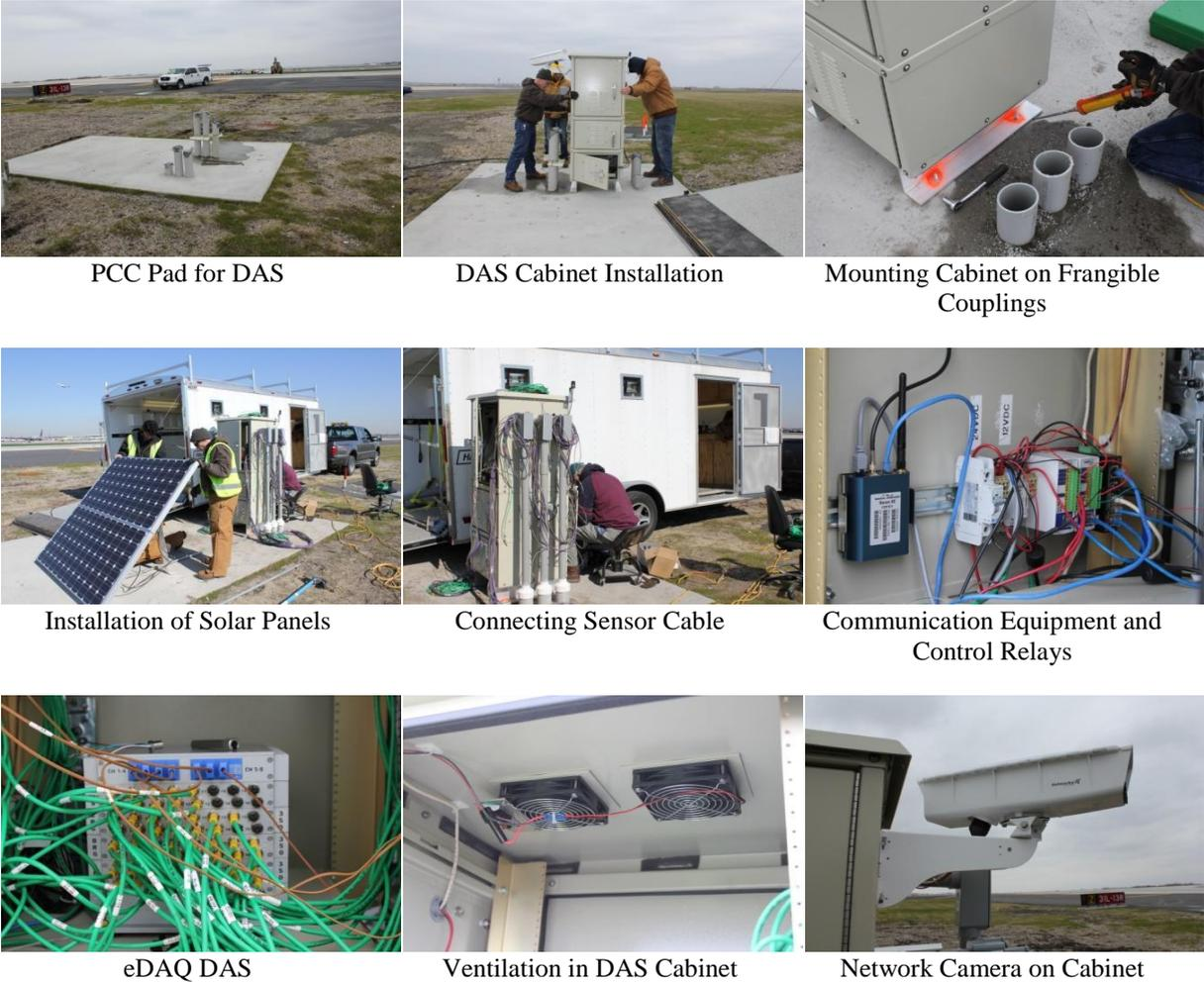
Figure 8: Installation of Data Acquisition System.
