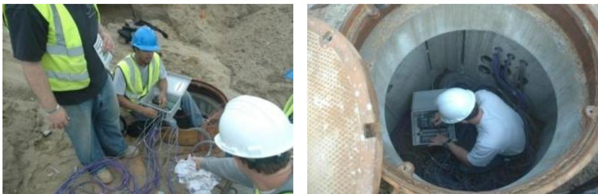
Figure 7: Installation of Data Logger to Collect Initial Instrumentation Data.
