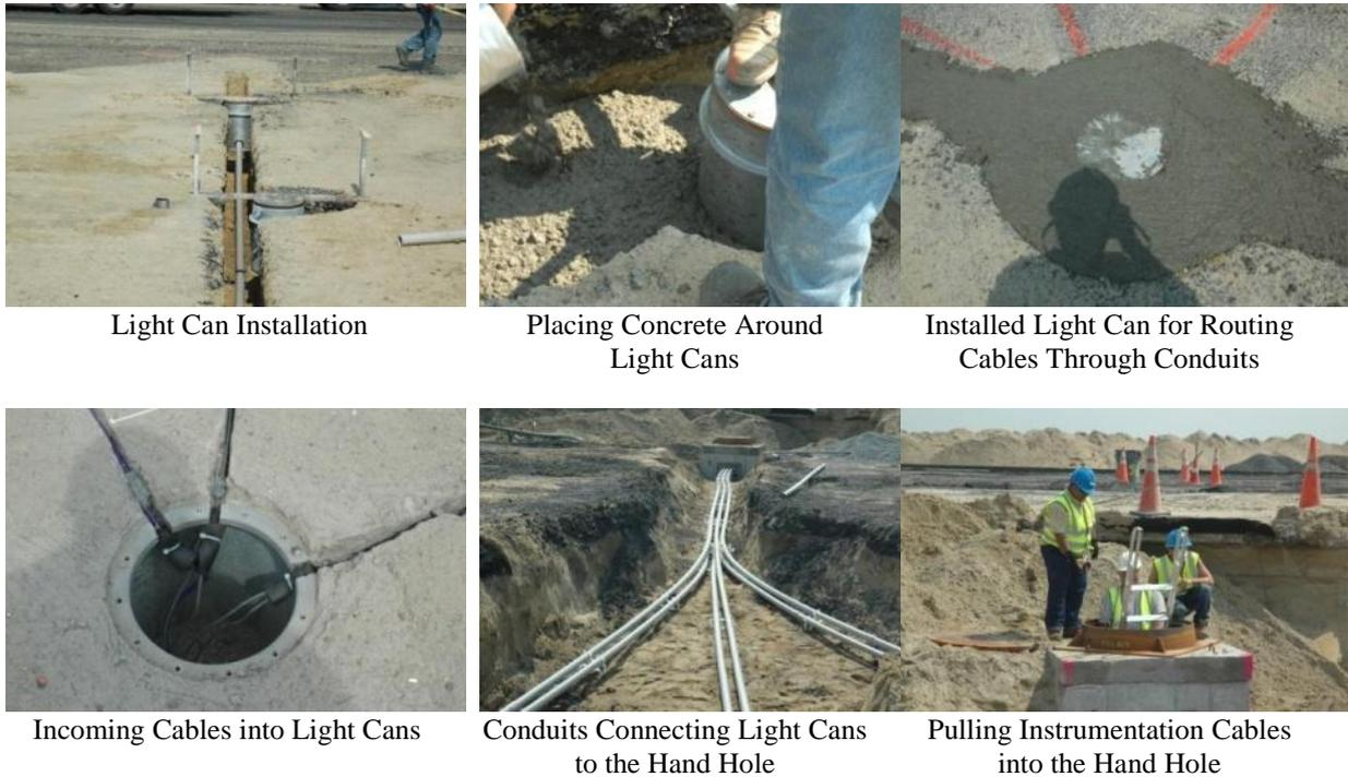
Figure 6: Routing Instrumentation Cables from PCC Slabs to a Hand Hole Located 150 feet (45.7 m) from Taxiway-Z Edge.
