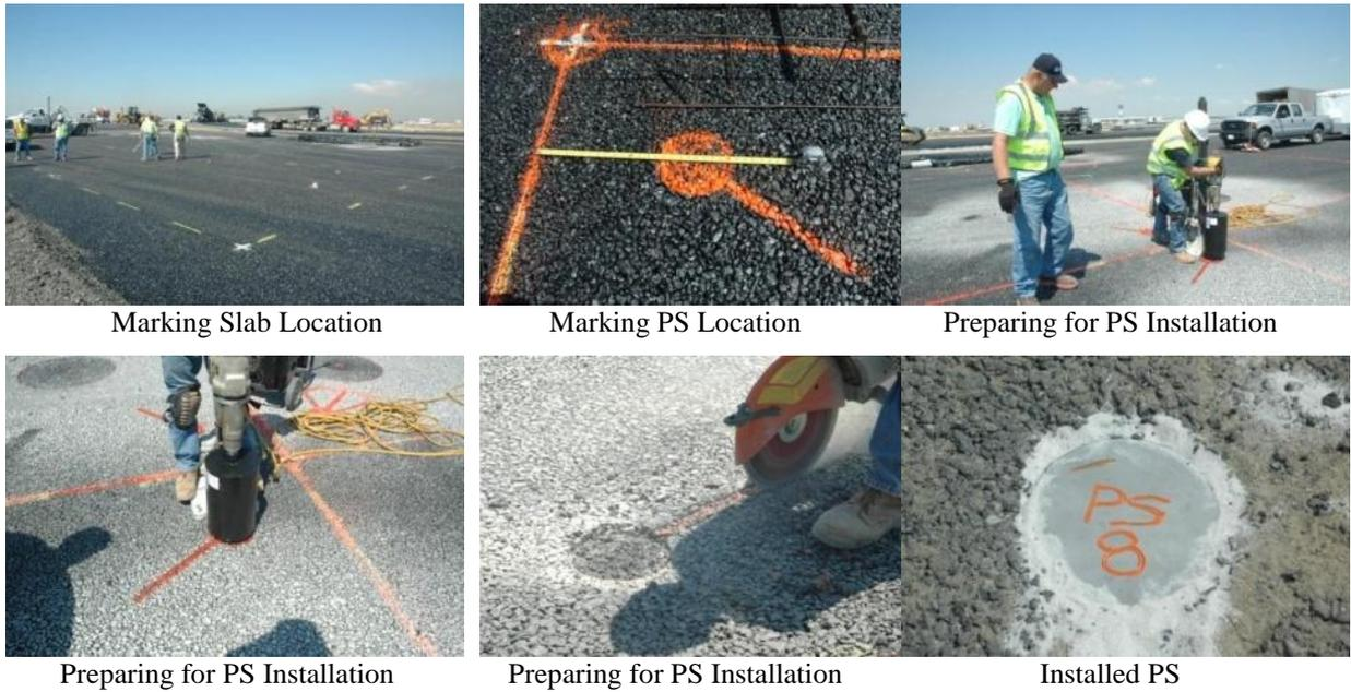
Figure 4: Installation of PS in Taxiway-Z pavement instrumentation project.
