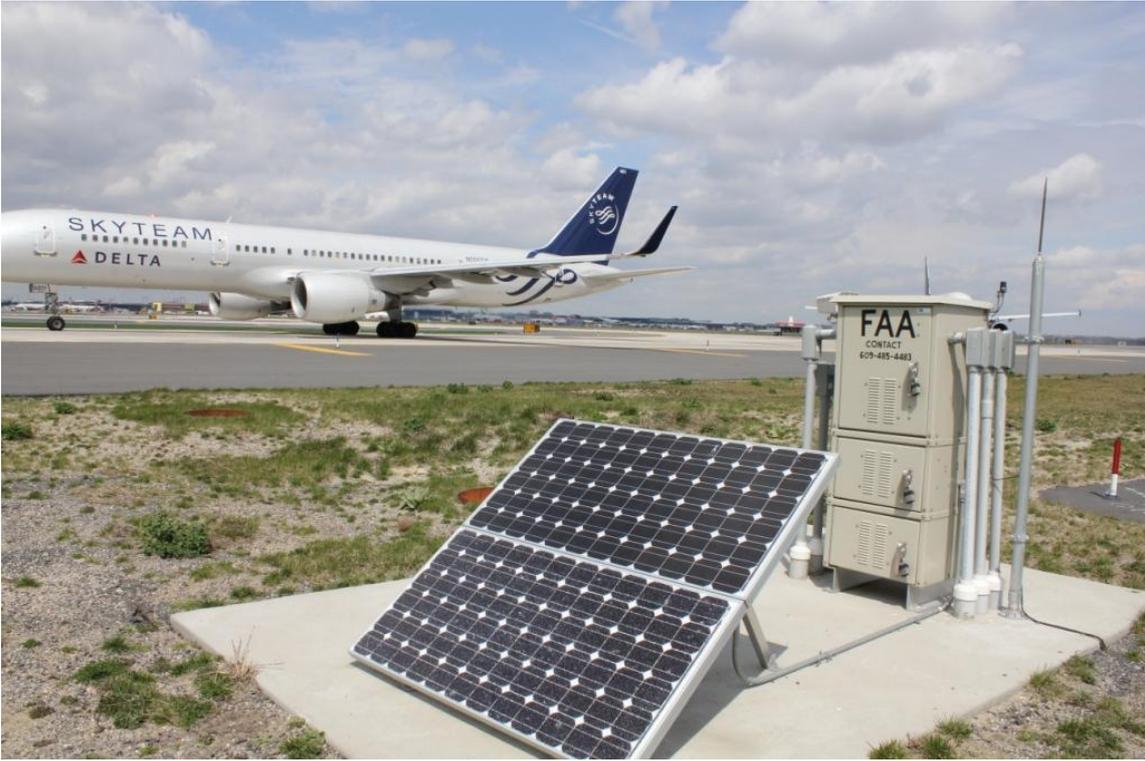
Figure 9: FAA Data Acquisition System at Taxiway-Z Pavement Instrumentation Project.
