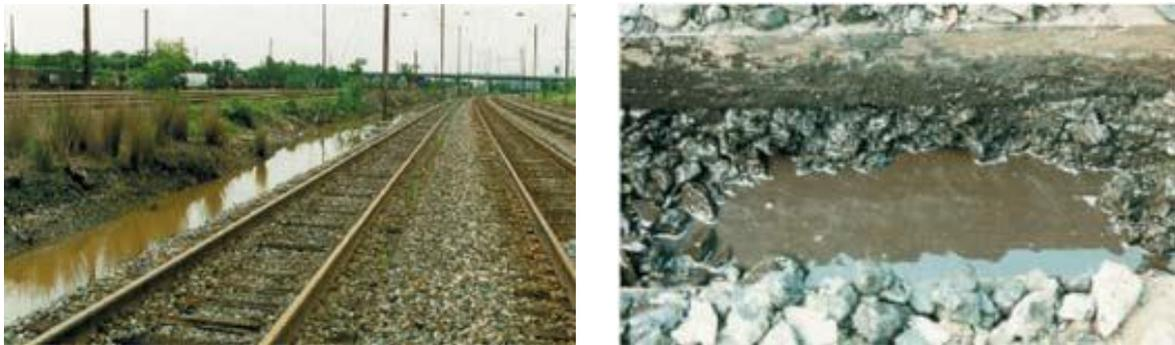
Figure 1: Tracks suffering from poor drainage (Adopted from Lackenby, 2006)
