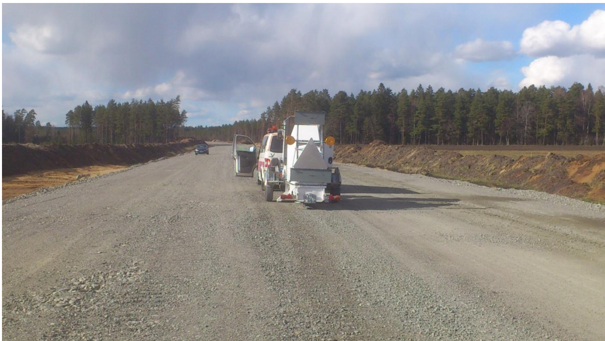
Figure 7. The subbase offered a fair surface for FWD testing in April 2012.
