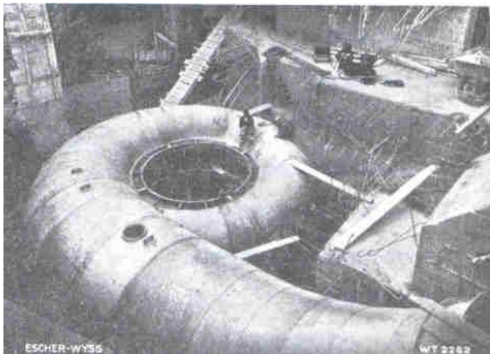
Fig. 8.3 Kaplan scroll casing of steel plates
