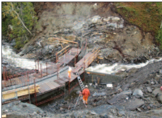
(a) Dam and intake structure for the Væla hydro plant.
