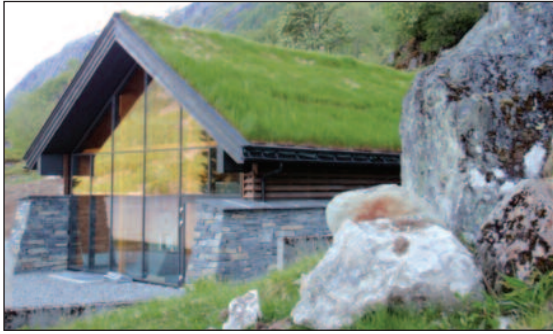
(c) A powerhouse for small hydro. Photo: Småkraft.
