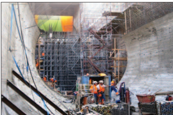
(f) Draft tube construction at Kongsvinger. Photo: Eidsiva Energi.
