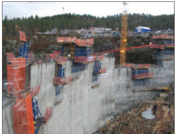
(g) Sarvsfossen dam during construction.
