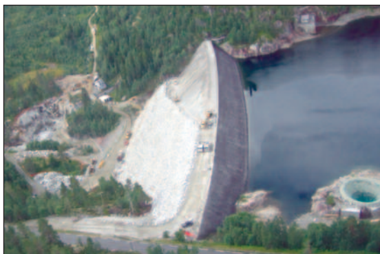
(l) The Venemo dam during upgrading. Photo: Statkraft.
