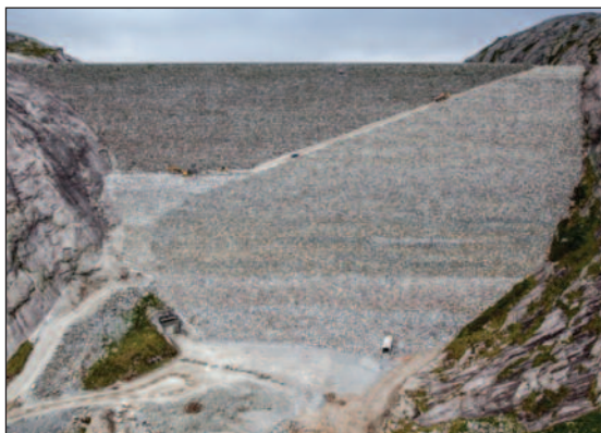
(m) The Svartevatn dam during upgrading. Photo: Sira-Kvina.
