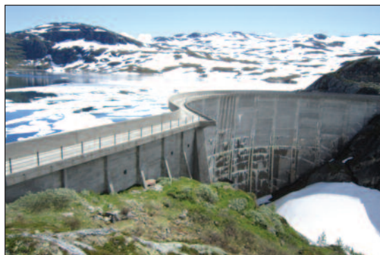
(n) The Votna arch dam. Photo: Hydro Energi.
