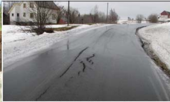
Wedge with insufficient inclining causing unacceptable uneven frost heave.
