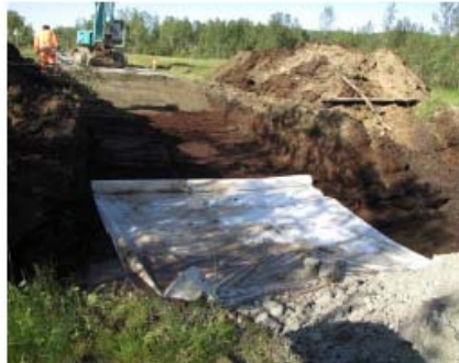
Construction of a wedge.
