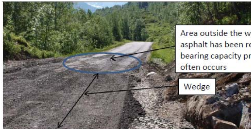
Wedge with insufficient inclining causing unacceptable uneven frost heave.
